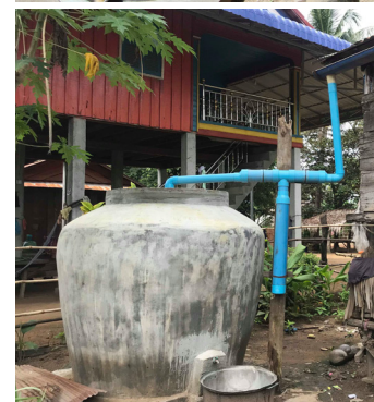
(Top) Concrete ring tank 3,000 litres (Bottom) Jumbo Jar 3,000 litres
