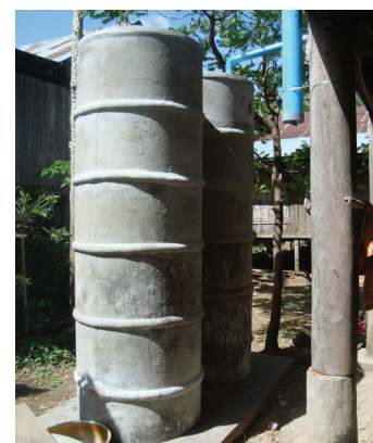
(Top) Ferro-cement tank 35,000L, (Middle) Elevated tank 14,000 litres, (bottom) Concrete ring tank 20,000 litres
